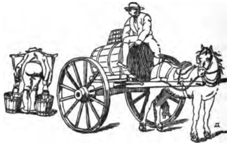
The Water Supply.
